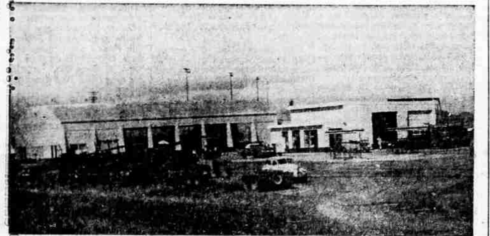
REPAIR SHOP, SERVICE STATION —This new facility for loggers, located at the state highway weighing station, adjoining the Veterans Administration's Memorial field on Crater Lake highway, will be opened in the fall, according to Steve Wilson, builder and manager, who transferred his operations from Trail last spring. —(Jerry Gamble Photo).
