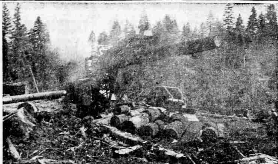
LOADING TRUCK — The diesel powered "heel boom" holds suspended a log that has been lifted from a deck in the forest. Tongs at the end of a cable grasp the log and hold
