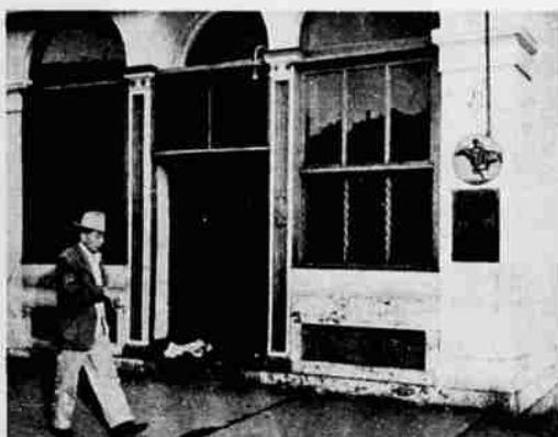
Long neglected, Pony Express depot will be restored.
