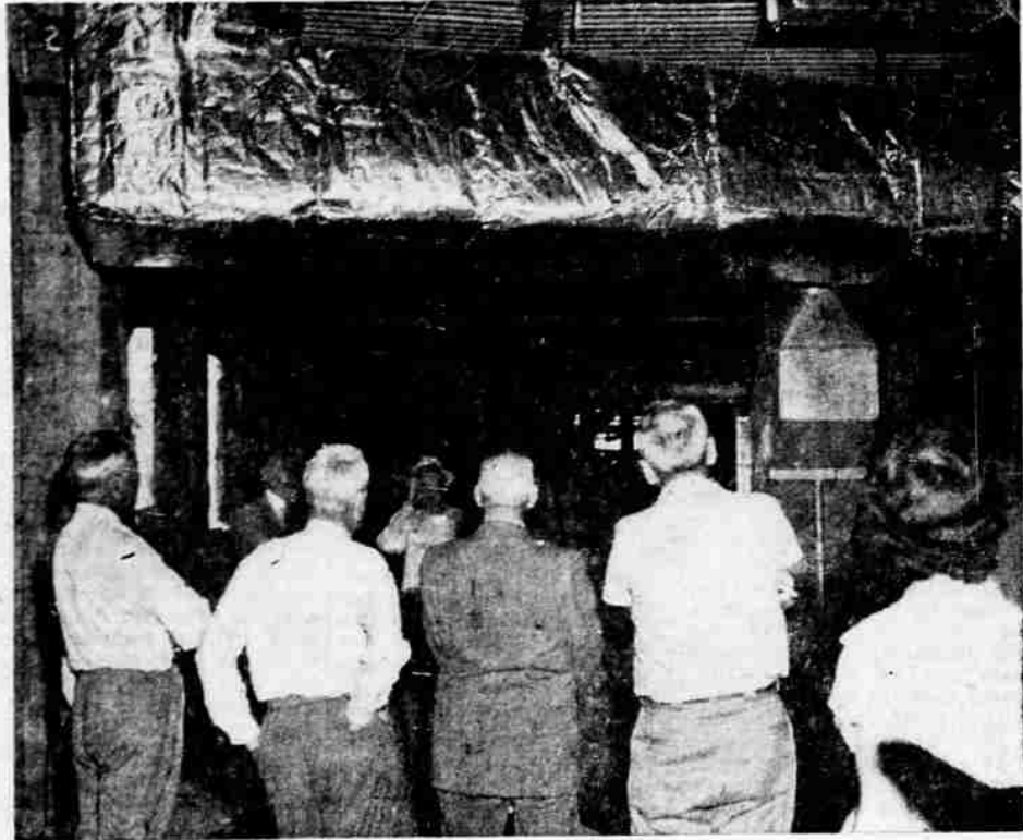
GUIDED TOUR — W. R. McCormick (hand in hat), clerk of the works for construction at Rogue Valley Memorial hospital, conducted a tour of members of the board of directors of the Jackson County Chamber of Commerce, through the big building last week. To the left is Otto J. Frohnmayer, of the hospital board. County Judge Rodney
