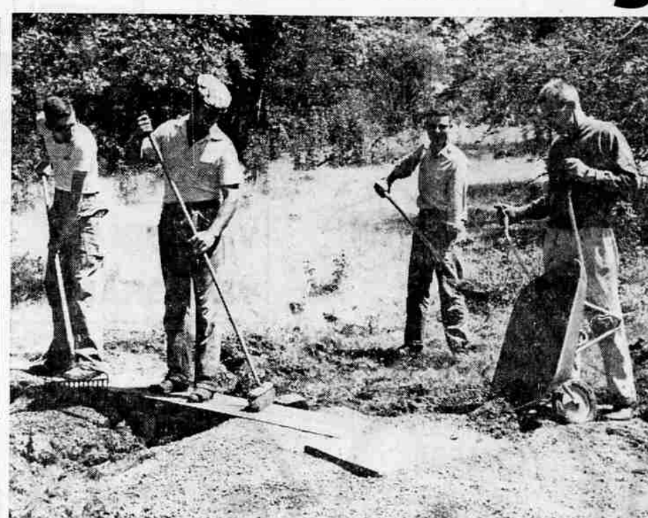
CLEAR PATHWAY —Four members of the Medford Junior Chamber of Commerce are shown repairing a small footbridge on a path to restrooms at Prescott park on Roxy Ann butte Sunday. They are, left to right, Al Holmes, Leonard Howe, Chuck Henry and Al Franzke. Another work-day has been scheduled by the Jaycees next Tuesday. —(Kenn Knackstedt photo).
