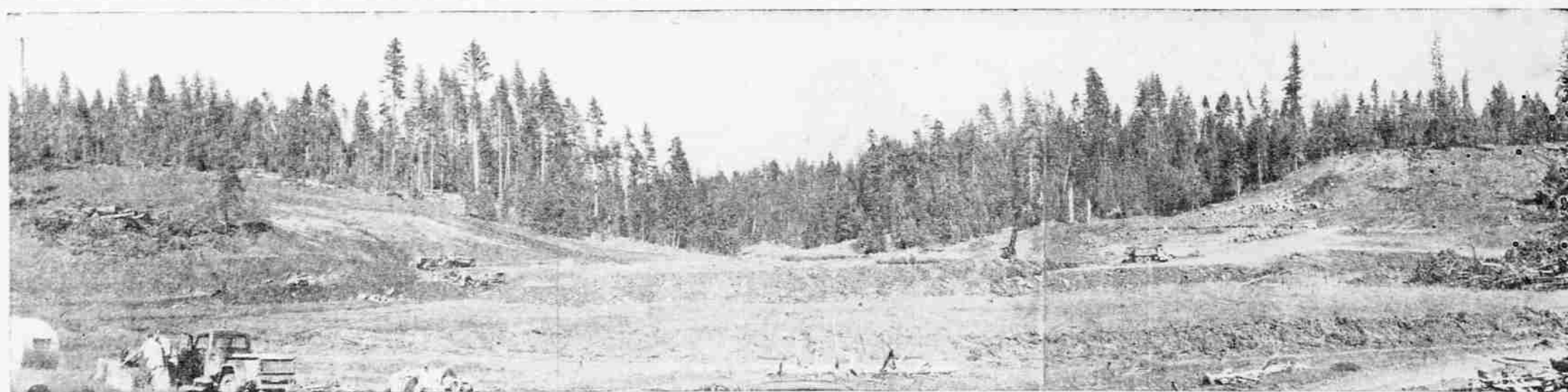
PANORAMA OF CONSTRUCTION SITE —The R. A. Heintz Construction company, Portland, is stripping the abutments on what will be the Howard Prairie dam, shown above. The Talent project dam will include 186,000 cubic yards of earth fill, 204,000 cubic yards of rock fill and a concrete core. It will be equipped with an outlet to the canal and a spillway. The structure, to be 1,000 feet across at the crest, 426 feet
