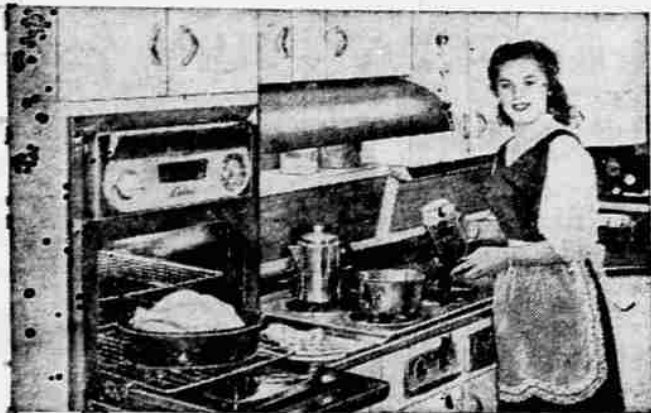
UP AND AWAY! —Ventilating hood installed above range area whisks cooking smoke, odors and grease to the outdoors before they have a chance to drift to other rooms of the house.
