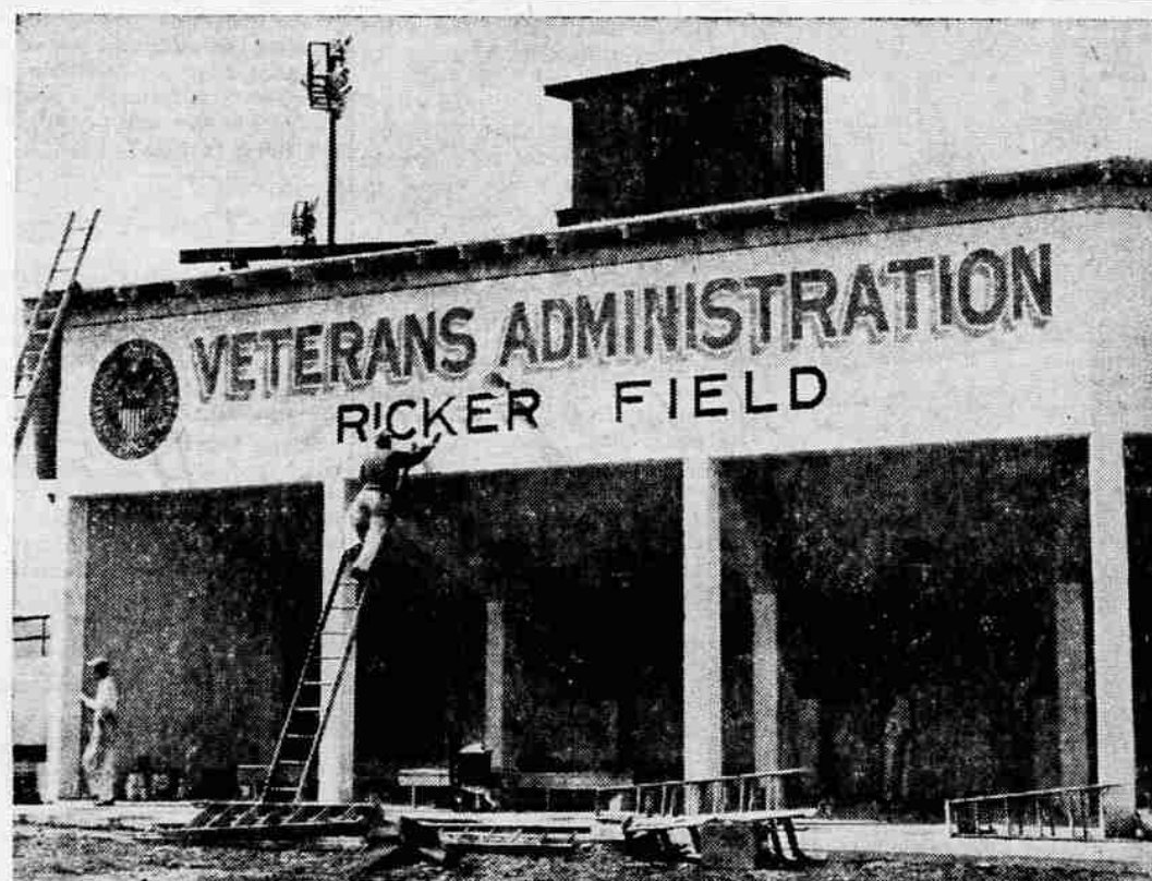
FINISHING TOUCHES —Above, a sign painter puts the finishing touches on the sign at the new stadium building at Camp White, while other workers clean up and complete last-minute jobs to get ready for dedication of the new structure next Thursday. The field was named after Eugene K. Ricker, manager of the Camp White VA Domiciliary. Highlight of the dedication ceremony will be laying of the cornerstone and an address by Ricker. The ceremony will be followed by a ball game between the Camp White team and Cheney Stude.
