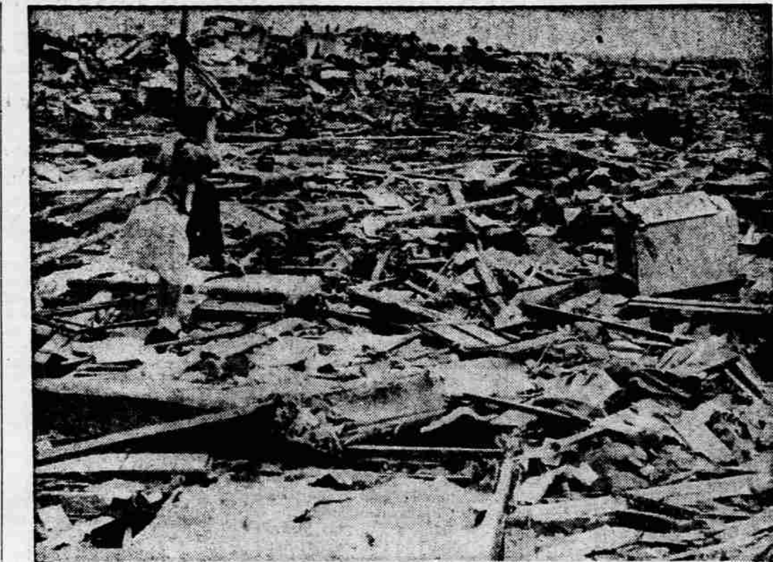
GONE! EVERYTHING IS GONE!—This unidentified woman nearly collapses as she views the rubble of her home in Ruskin Heights, Mo., after a tornado leveled it and
