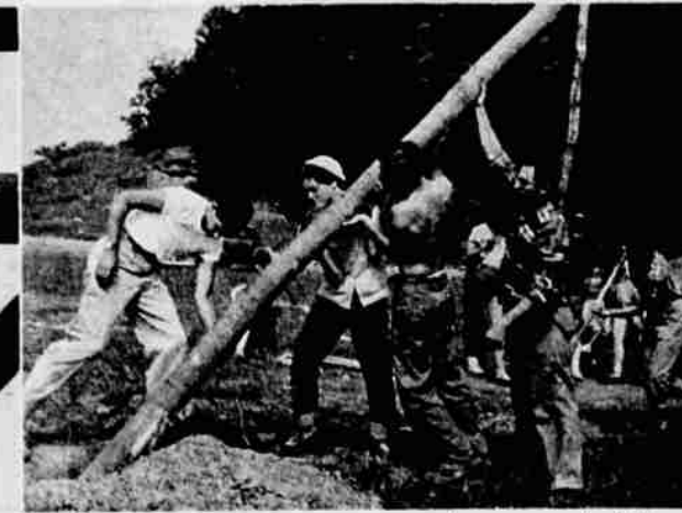
Putting up a pole to carry power to a camp building, youngsters learn to work together to get a job done.
