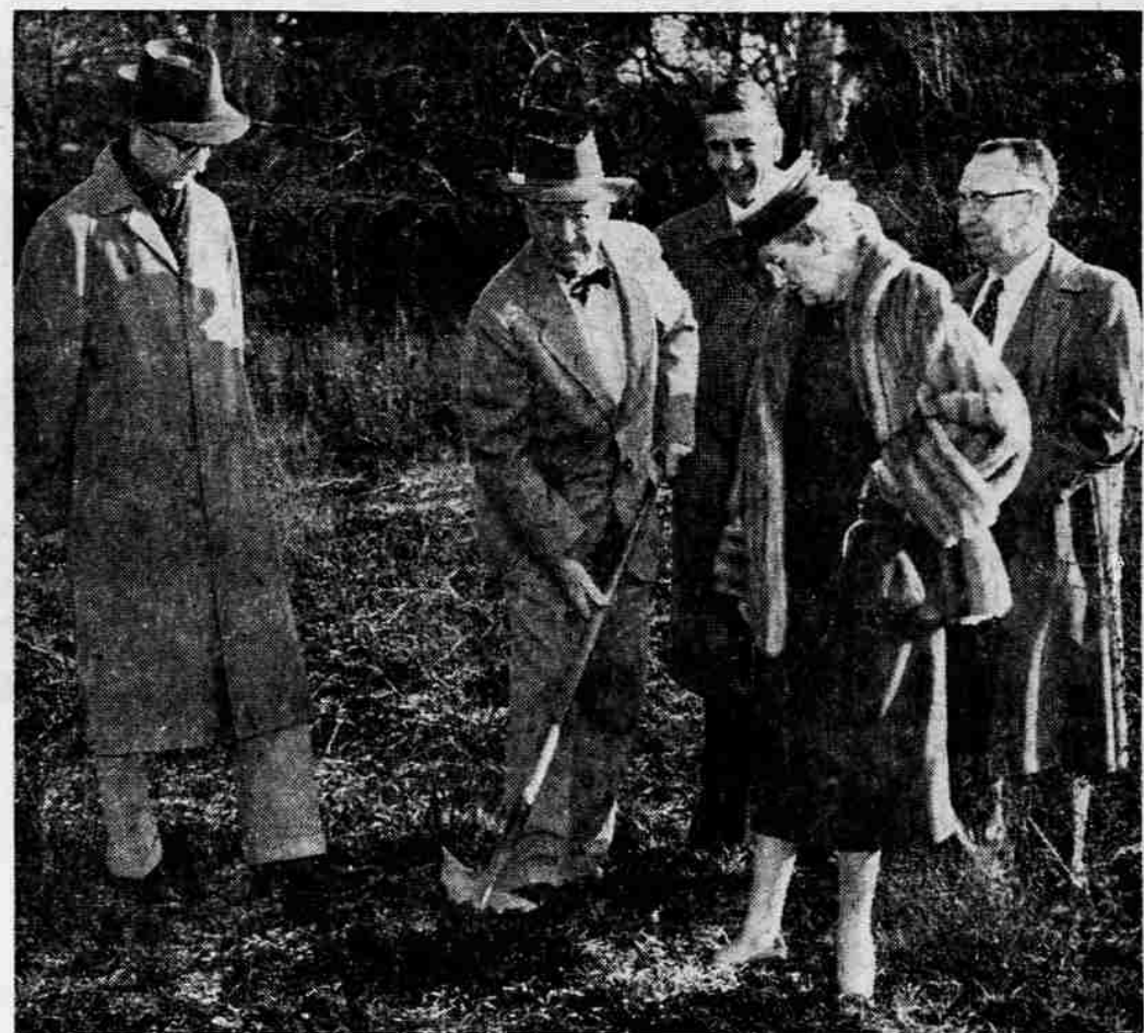
GROUND BREAKING —A. S. V. Carpenter lifted the first shovelful of dirt last Wednesday in preparation for construction of the new Red Cross chapter house near Hawthorne park. The building and site are a gift to the local chapter from Mr. and Mrs. Carpenter. Others attending ground breaking
