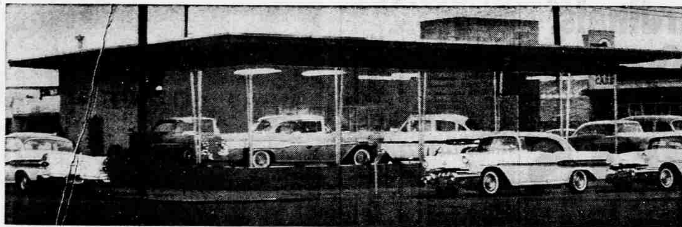
NEW SHOWROOM —Shown above is the new Dean and Taylor Pontiac company showroom at Sixth and Grape sts., Medford, construction of which recently was completed. The showroom is the final phase of development of the company lot to be completed in a series of projects since 1940. The
