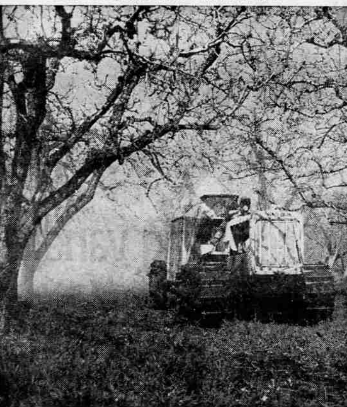
SPRAY OPERATIONS —Dusting operations were progressing more normally than early spray operations, which necessitated as many as three tractors to pull heavy spray rigs loaded with liquids. Some orchardists reported difficulty in even getting lighter dusting units, like the one shown above, through low areas. With better weather and good drainage, many of the orchards will be back on schedule next week.
