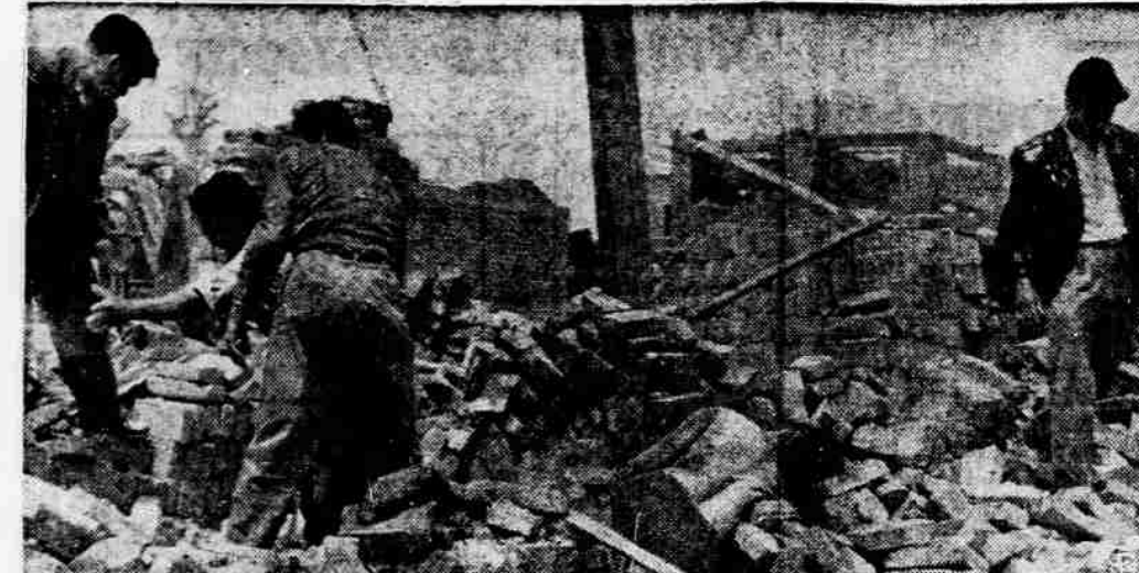
DIGGING THROUGH RUBBLE after two explosions razed Mexico City fireworks factory, rescue workers seek victims of blast which killed at least 11, left 100 injured. (Note body of victim at center. Windows one mile distant were shattered. (International)
