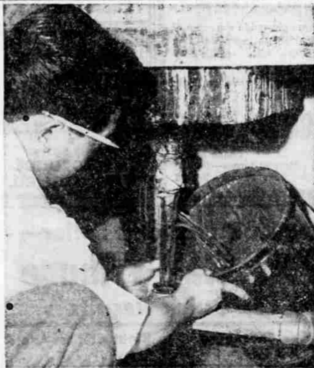
QUAKE ROCKS SAN FRANCISCO BAY AREA —Water gushes from a ruptured drain pipe in United Press photo darkroom in the San Francisco News building following a sharp earthquake which was described as the worst to hit the area since the disastrous 1906 quake and fire. Above, Max Gutierrez presses all the available buckets into service until the water can be shut off.
