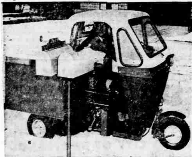
MAIL GOES THROUGH IN COMFORT—Newest motorized vehicle for the U. S. Post Office is this "Mailster." The sleek, maneuverable machine is designed for fast, efficient and economical delivery of mail and parcel post in residential areas now being serviced by carriers on foot or bicycle. The Government has ordered 1500 of them from Cushman Motor Works in Lincoln, Neb. They will be used by post offices in the Southeast, Southwest and in California.
