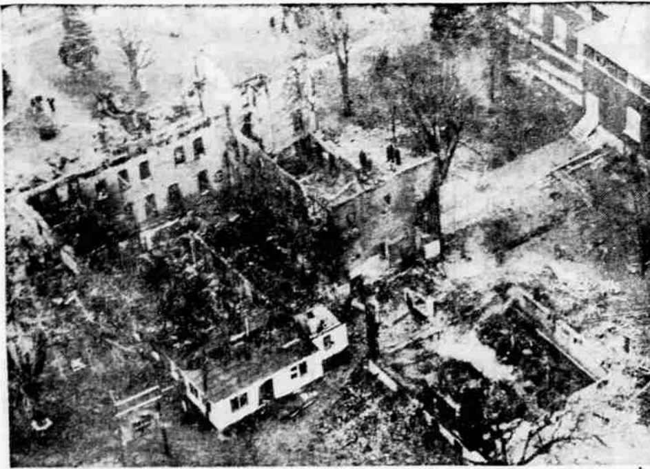
71 DIE IN HOLOCAUST—Fire-blackened walls are all that remain of the Katie Jane Memorial Home for the aged in Warrenton, Mo., after an explosion and fire mushroomed through the building killing 71 persons. Authorities said more than 225 persons, including patients and visitors, were in the building when the fire started.
