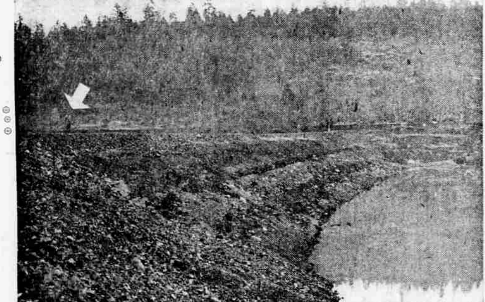
HIGHEST EARTH FILLED DAM —This is Jackson county's highest earth-filled dam, standing 84 feet high from its base. Arrow points to its owner and contractor, Robert von der Hellen, Eagle Point. His plan for the dam, which has a storage capacity of 900 acre feet of water, is to irrigate 300 acres of land in the Eagle Point area where he intends to harvest 150 acres each of pears and clover. Von der Hellen and three men completed the structure last fall after three and a half months of work.
