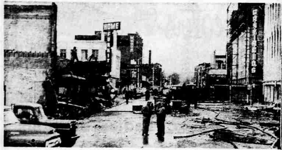
CLEAN UP JOB STARTS—Looking north on Virginia street in Reno, Nevada, the scene takes on the aspect of a war-torn city the day after gas explosions rocked the downtown business section. Completely destroyed building at left was Paterson Department store. Three buildings were destroyed and a score of others were damaged. Two persons were killed and 42 others were injured.
