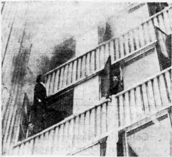
PRECARIOUS PERCH —Roy Tietjen stands on window-sill of sixth floor of Northward Building in Fairbanks, Alaska, shouting to persons trapped on the two floors above him to "stay put." More than 200 persons were trapped on the upper floors of the building as the result of smoke and fire in a lower floor television studio. One man was killed and nine persons were injured.
