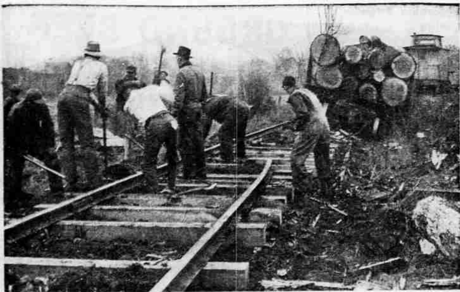
ON AGAIN —The Medford Corporation logging train, which runs between Butte Falls and Medford, was on time this morning after repair crews made quick work of relaying the 100 feet of track torn up when five cars of the 30 car train were derailed early Thursday morning. This particular section of track, just south of the Little Butte creek trestle, has been the scene of three derailings in the last four years. Workmen, above, had only one car to place back on the track when the picture was taken just before noon yesterday.
