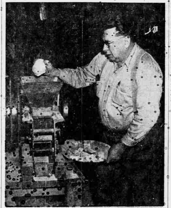
JAW CRUSHER —In order to break chunks of mineral bearing rock into smaller pieces for processing, Joe McCulley puts them through this jaw crusher he rigged up himself from odd pieces of machinery. Broken pieces fall into the pan beneath the receiving bin. The ore is ground still finer with a mortar and pestle before going into the ball mill which, when water is added, beats the rock into a sloppy mixture.
