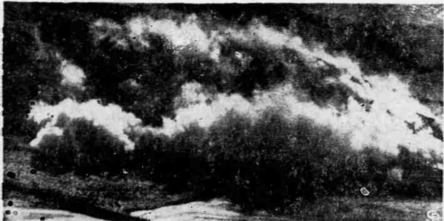
BLOWING UP MOUNTAIN , 600,000 pounds of dynamite blasts rock for Southern Pacific's new railroad causeway, one of history's largest non-atomic blasts. (International)
