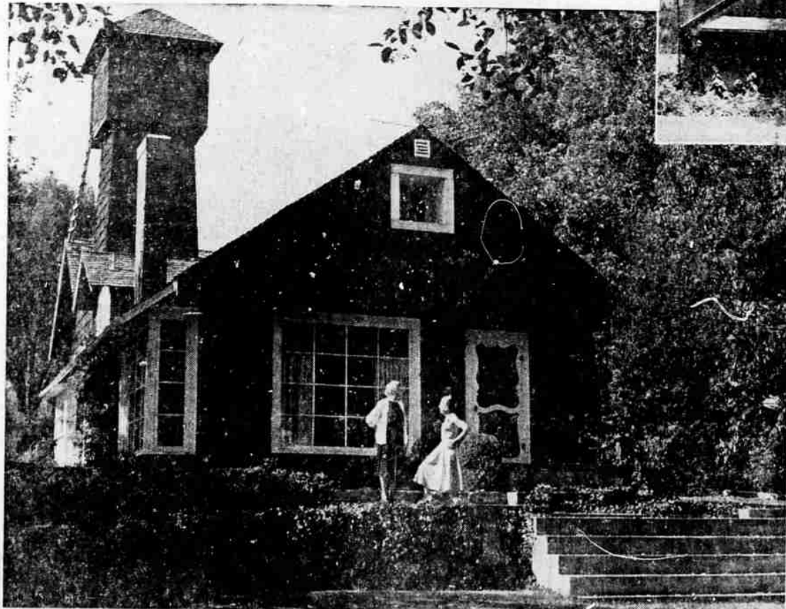
Mr. and Mrs. Lester Adams and Mrs. Adams' mother, Mrs. Guy Flenner, spent 13 years transforming an ordinary farm house (see inset) into this charming, comfortable home. The exterior is of shake, board and batten, painted maroon and white; water tower provides interest.
