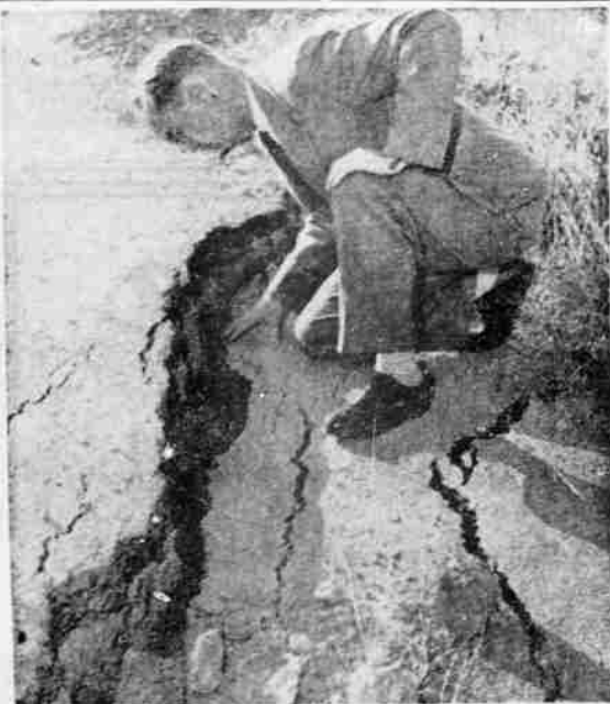
SLIPPING EARTH MENACES more than 300 homes in the Palos Verdes section of Los Angeles. The crack is two-and-a-half miles long. No immediate reason was discovered in an emergency meeting of engineers. An unidentified man examines crack. (International Soundphoto)
