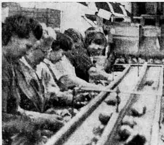
SORTING LINE —Pears are sorted on conveyor belts as shown above at the Myron Root and Company plant. In this process, the defective fruit is discarded and higher quality pears are sent on for sizing. The fruit is separated into grades according to size. Later, the pears are packed into boxes.
