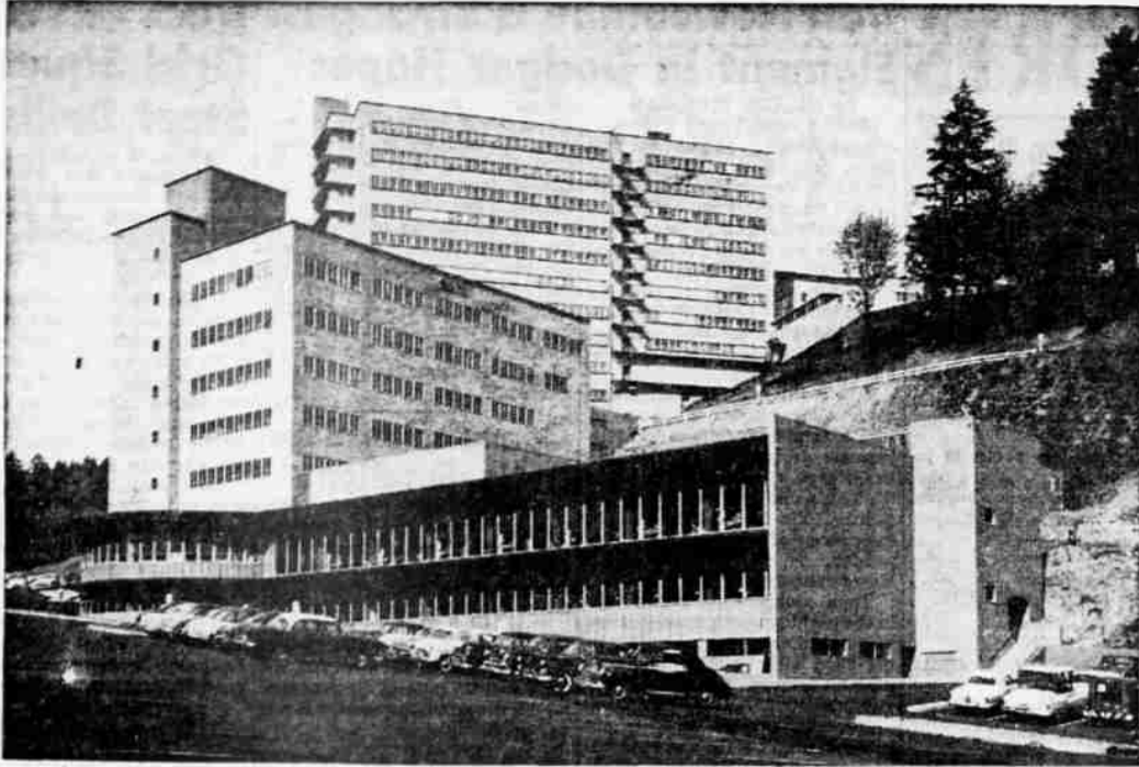
DEDICATION NEAR—New building of the Dental school of the University of Oregon, under construction since July, 1954, will be dedicated Sept. 14. Structure is located in the university's medical center in Sam Jackson park, Portland.
