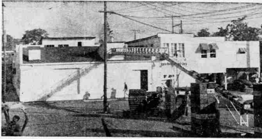
IN MORNING SUN —This is the front of the processing plant facing on 13th st. as it looks in the early morning sun. In the foreground lot empty boxes coming from inside the plant
