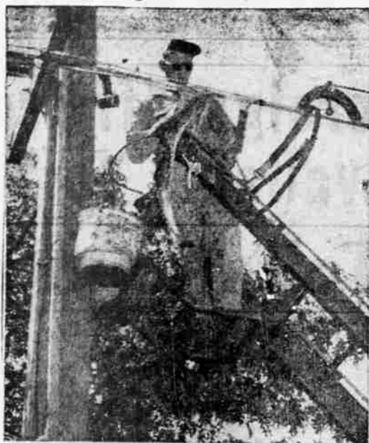
AUTOMATIC LADDER —A device such as this automatic ladder would be ideal during pear picking season. Pacific Telephone has several such rigs in this area for jobs such as this one. Splicer Gene Rosencrans is splicing cable together along Hillcrest rd.
