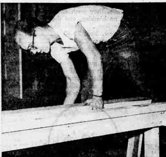
BUILDING BENCH — Bill Walker, student minister at First Methodist church and chairman of Amigos Internacional, concentrates on the building of a bench at the work night Thursday evening. Before using all the lumber that was donated by the Elk Lumber company, the group completed six benches.
