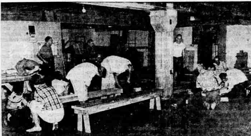
BENCHES BUILT — Amigos Internacional, a group of people in the community interested in the Mexican nationals, gathered at the First Methodist church Thursday for work night. Armed with an assortment of tools the group built benches for the barracks grounds where Mexican laborers live. Other work night sessions are being planned. The group is trying to locate a place in Medford that could be used as a service center, where translators would be available for the Mexicans where they may relax and find help in routine daily matters. (Brainard photos)
