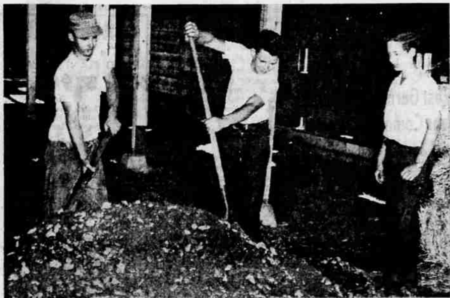
PREPARING FOR FAIR —There's lots of cleaning and repair work to be done before the annual 4-H and FFA fair gets under way Tuesday. Above: Galen Clifford, left, and Jack Esp, center, spread gravel from a road through one of the main shelters at the fairgrounds. David Hughes supervises at right. All three boys are members of the Eagle Point High School Future Farmers of America chapter.
