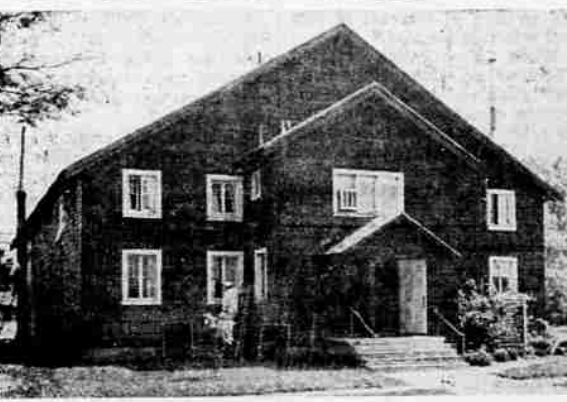
CENTRAL CHURCH OF CHRIST Gets First Coat of Paint
