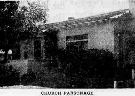
CHURCH PARSONAGE 523 North Bartlett Street
