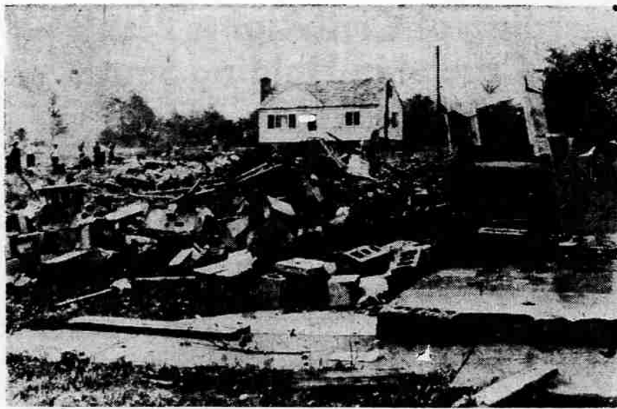
GONE WITH THE WIND —The home of John Reapsommer is a mass of rubble after it was leveled by a tornado which struck Girard, O. Living in the basement for six years while the house was being completed, Reapsommer, his wife and three children were not injured. They were to move upstairs in a week.
