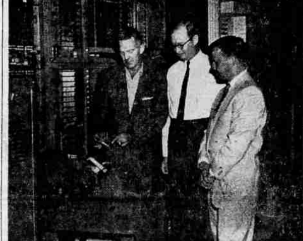
CHECK TOLL TICKET — Fred E. McGrady, left, chief sales engineer, Pacific division of Stromberg-Carlson company, checks the toll ticket recording equipment at Columbia Utilities company's White City central office with John W. Kirby, center, vice president of Columbia; and Ernest D. Larson, Oregon representative of Stromberg-Carlson. The new equipment enables direct distance dialing and is the fourth such installation west of the Mississippi.
