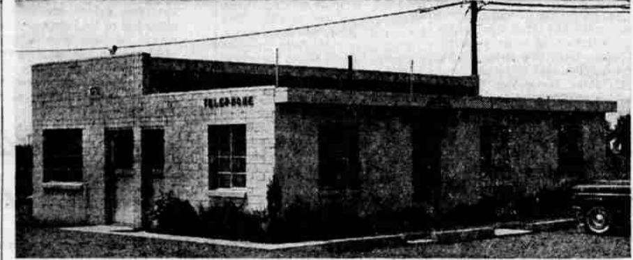
CENTRAL OFFICE—Telephone toll-ticketing equipment recently was installed at the Columbia Utilities company's central office in White City, above, enabling direct dialing for White City, Eagle Point, Shady Cove, Prospect and Butte Falls subscribers. The change over to the new system is the first in the state.
