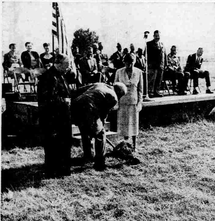
CONSTRUCTION STARTS —Ground was broken this morning for construction of the $2,000,000 Rogue Valley Memorial hospital. In the picture above, Alfred S. V. Carpenter, one of the major donors for the hospital, is shown turning the first shovelful of soil, watched by Mrs. Carpenter and the Rt. Rev. Benjamin Dagwell, bishop of the Episcopal diocese of Oregon and head of the hospital
