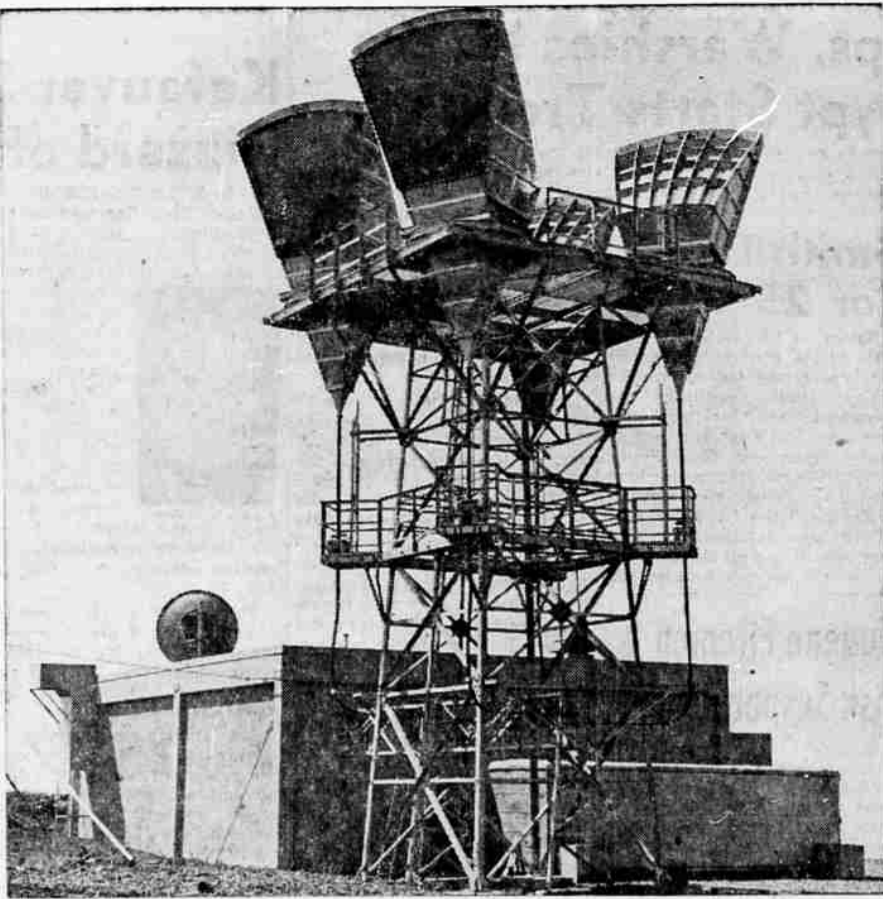
MICROWAVE ANTENNA — Pacific Telephone and Telegraph company's new microwave relay station on top of Baldy mountain, southeast of Medford, was put into operation at midnight last night. It was the last link in the company's San Diego-to-Seattle system
