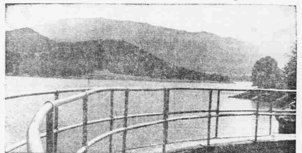
LAKE TO RISE FROM HERE —This view is taken from the top of the existing concrete arch dam which backs up Emigrant lake. The present dam will serve as the core of a new earth-fill dam, which will rise about 84 feet
