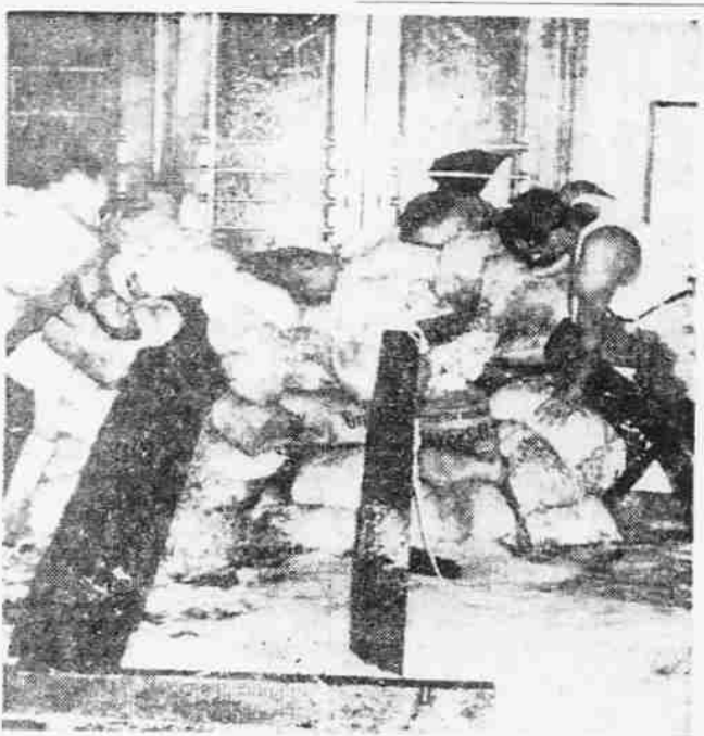
SUBWAY SUBMERGED—Workmen struggle to shore up doors at the Eighth Street subway station in New York in vain effort to stem the onslaught of water pouring into the subway arteries as a result of the 25-hour fire at the nearby Wanamaker Department Store building. The torrents of water thrown on the building by firemen cascaded into two arteries of the city's subway system, causing the worst commuter snarl in New York's history. —NEA Telephone
