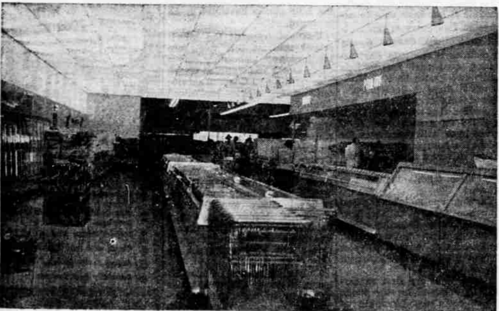
NEW ADDITION—This 48 by 110-foot addition to the Big Y contains meat, frozen foods, dairy products and beverage departments as well as a branch of Swem's Record store and the Big Y appliance store. The expansion and modernization program was inspired by the store's strong need for more space.
