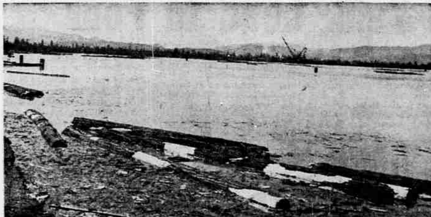
NEW MILL POND —Located west of the Crater Lake highway and northeast of the airport is a new Medford Corporation mill pond. Crews have been working on the pond for several months. Company officials have so far declined to announce details on the project.
