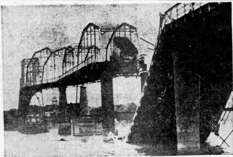
IOWA BRIDGE IS FALLING DOWN —Two drivers thank their lucky stars they escaped death or injury in this spectacular collapse of a section of bridge spanning the Mississippi River at Muscatine, Iowa. The trailer of one semi trailer precariously, spilling its load into the river. The cab of the second truck went into the water. Collapse of the bridge followed an earlier auto accident that weakened main girder of the bridge.
