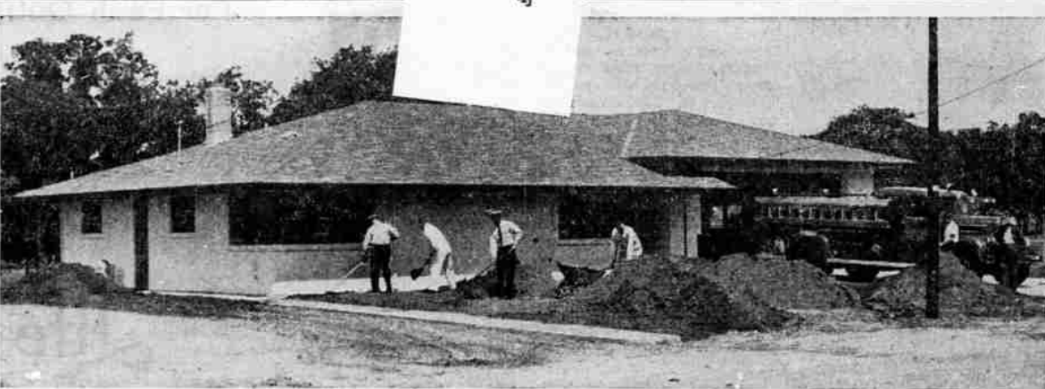
NEW FIRE STATION—Firemen are shown spreading top soil preparatory to landscaping around the new east side Medford fire station. The fire hall, at 530 Highland dr., was occupied last week and an open house was held Sunday afternoon with
