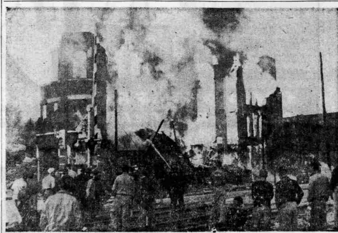
FLAMING INFERNO —Ten persons died and five others were injured when a gas explosion demolished a three-story building Friday in Pulaski, Va. The 10th victim was pulled from the debris Friday night before police began the task of identification. One of the injured was in critical condition, and two others were listed as serious. The explosion was touched off when W. J. McHaffey, a 75-year-old cafe owner, struck a match to start a gas water heater on the first floor.
