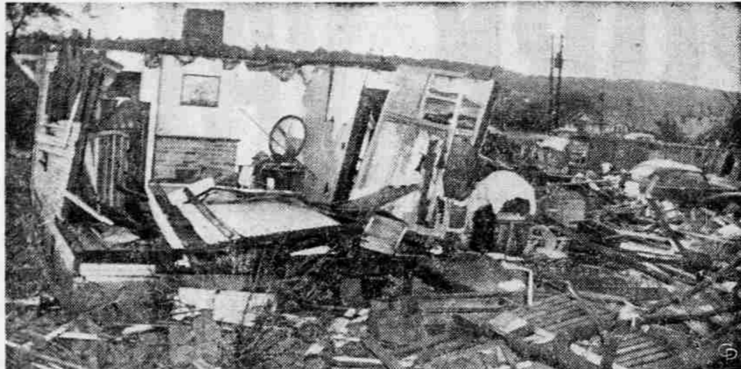
RIPPING THROUGH RURAL AREAS on industrial outskirts of Birmingham, Ala., tornado kills at least 17 persons, injures more than 200. This is one of numerous demolished houses, surrounded by debris ripped up by high winds. (International)
