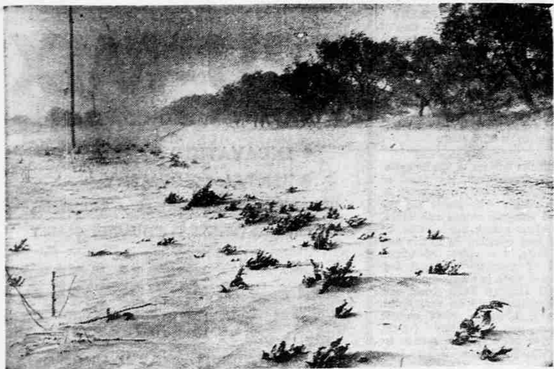
BURYING ROADS, DITCHES under sand, "worst dust storm in history" sweeps Snyder-Lamesa-Midland-San Angelo area in Texas. Shelter-belt of trees, planted during New Deal era, fails to hold back sand drifts covering roads, ditches. (International)
