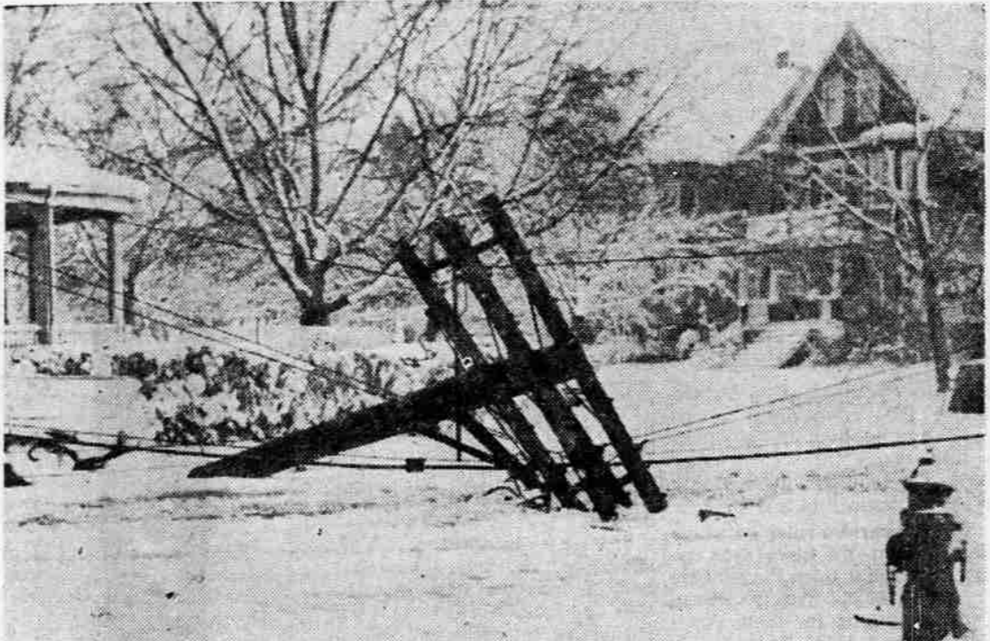
FREAK STORM —This scene at Somerville, Mass. is typical in many New England towns as recent heavy snows caused collapse of hundreds of utility poles, causing power failure and the danger of live wires in the streets.
