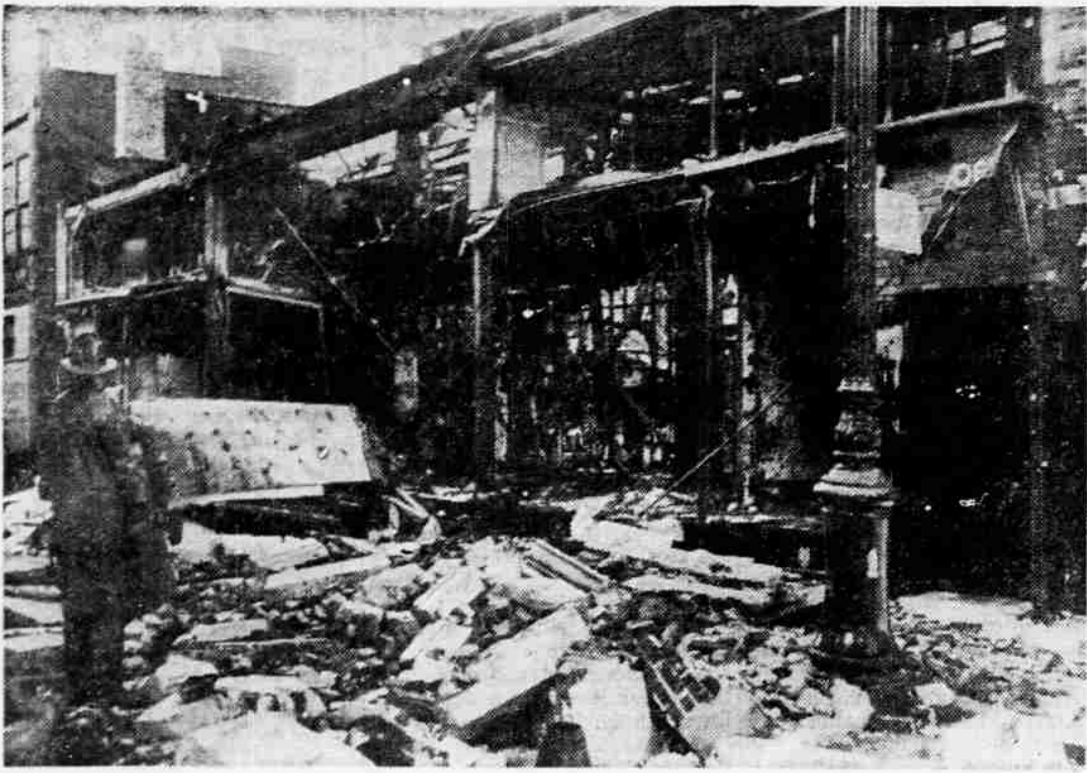
WHERE FIREFIGHTERS PERISHED —New York firemen look over the scene where six of their fellow firefighters were killed when the marquee and wall from a one-time theater fell on them. The building was being used as an artificial flower factory. Five other firemen were injured in the mishap. It was the largest toll of firemen lost battling a blaze in New York since 1932, when eight were killed.
