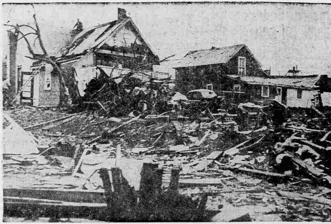
IN THE WAKE OF THE WIND —Homeowners at Marion, Ind., returned to this scene of desolation and ruin to begin the discouraging task of clearing away debris, patching roofs and rebuilding houses. Several persons in these two houses were injured when the tornado struck. One person in Marion was killed.
