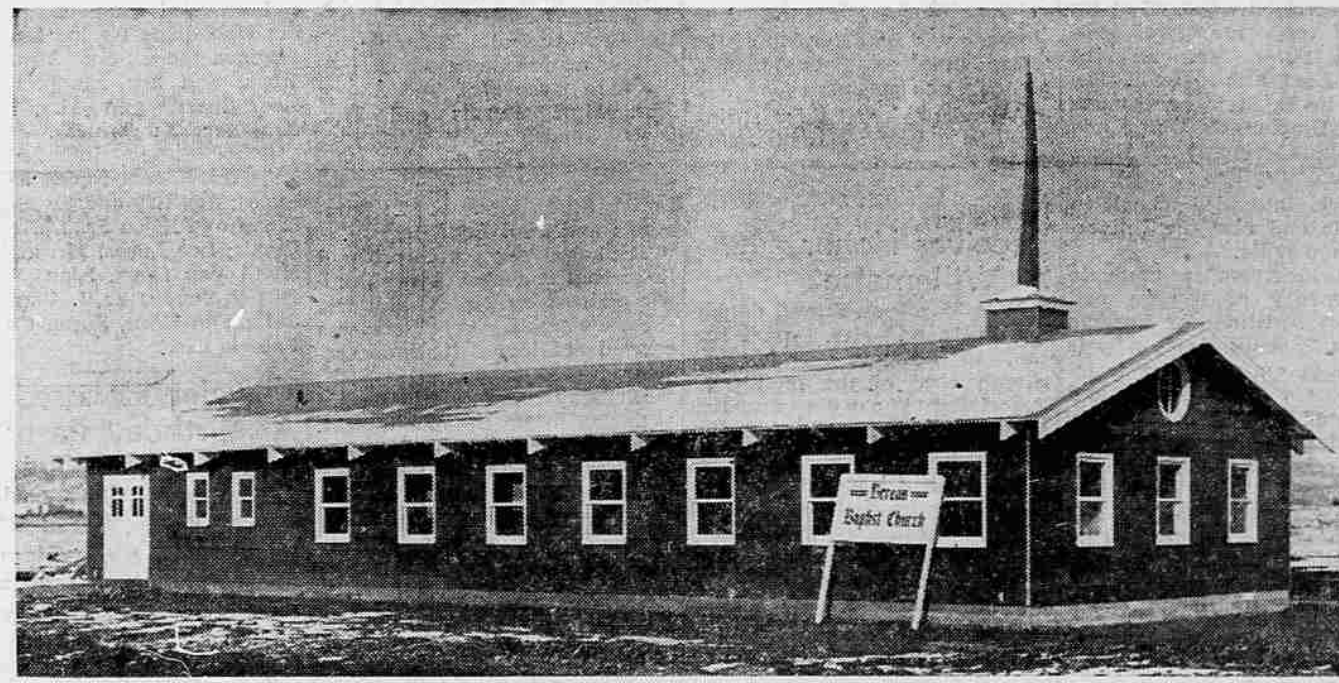
This new structure was erected by Berean Baptist church, White City, in recent months, with much of the work being done by members of the congregation. The exterior of the chapel is of redwood, with white paint trim. The interior will be completed in the near future, and dedication ceremonies will be held in about a month, according to the Rev. Glenn S. Wade, pastor. The church seats about 100 persons. The land for the church was donated to the congregation by Glenn L. Jackson of Medford.
