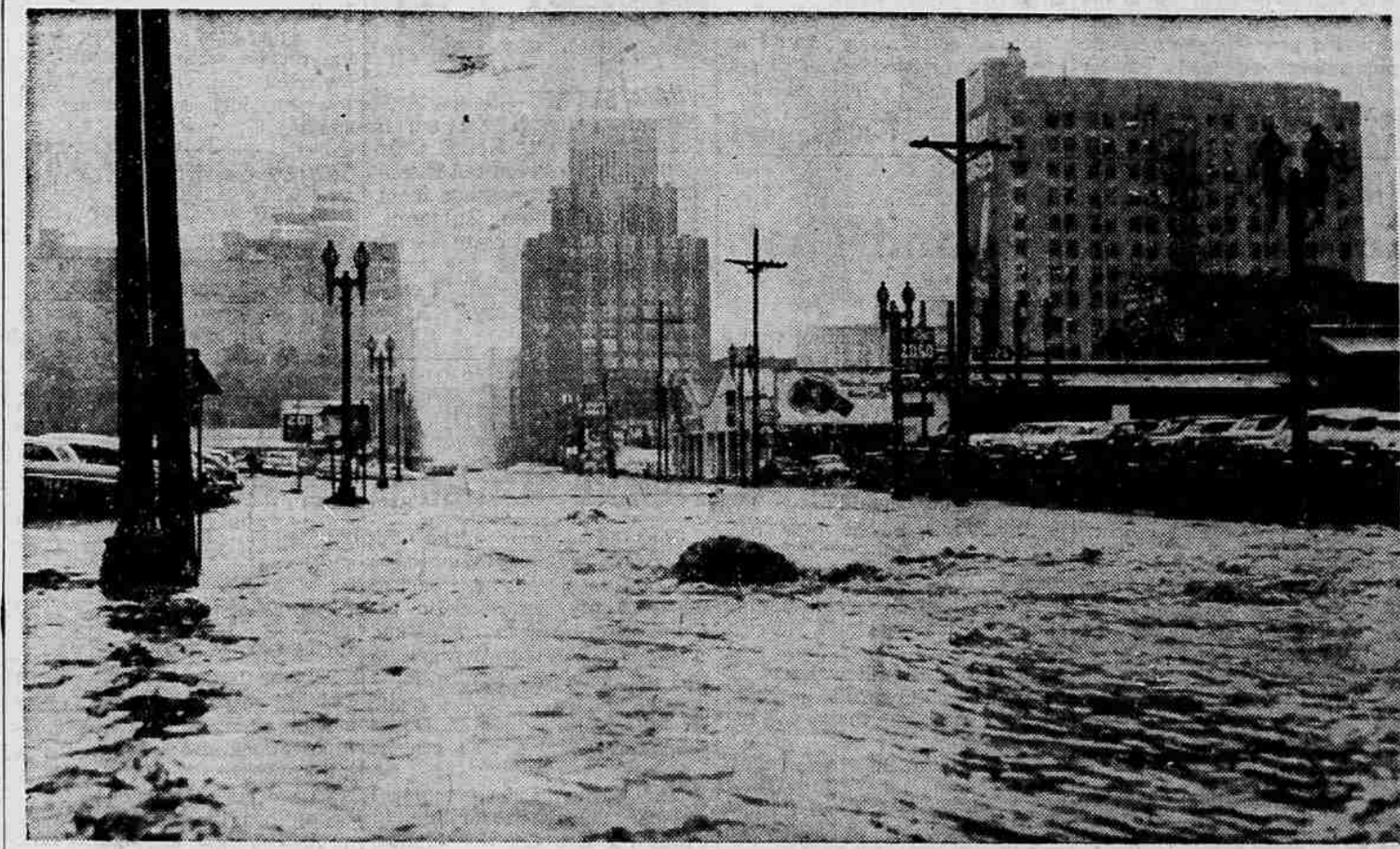
EVEN LOS ANGELES GETS FLOODED — Traffic is non-existent on Flower st. in Los Angeles after the main thoroughfare is turned into a river by the seven inches of rain that pelted Southern California. Manhole in center bubbles over with more water. Property damage was estimated at over a million dollars.
